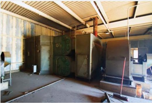
When Project Manager, Wes Maka, arrived on the scene for his estimate, he determined that even though it was possible for the units to be repaired, the cost of the repairs was almost the same as installing a completely new system. Combine that with the rapidly declining energy efficiency of the old units and replacement became a far better option and the clear choice. From 60% efficiency to 92% efficiency, Sterling Lumber was prepped for significant energy savings.
