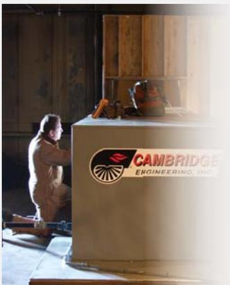
The four Cambridge units were a different story. Each was to be housed within shelters atop the roof, indoors, with no entrance wide enough to fit the sizable units. The conventional crane method could not be used in this situation. Instead, the 1,600lb units were lifted into the shelter by a pulley system designed by the Four Seasons team. The units were raised through bombshelter doors within each rooftop shelter, and once inside, a second pulley system moved these units into place.
